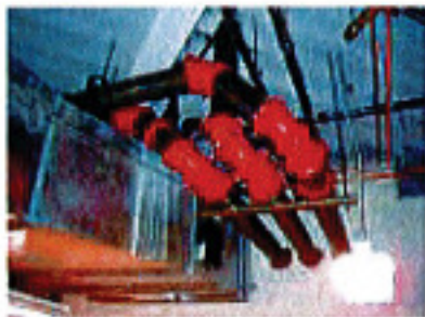
Figure 1 - The heavy pipe and short radius elbows shown in this photo had to be removed and replaced with material for a beverage chase at considerable cost.
